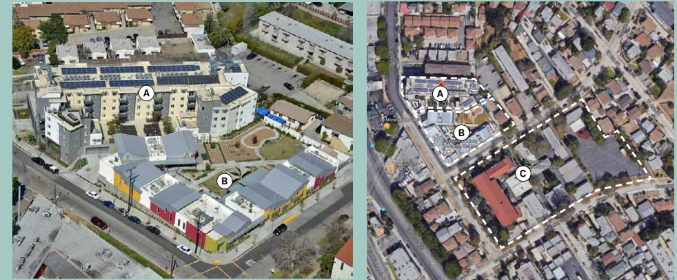
A RIO VISTA APARTMENTS B GLASSELL PARK EARLY EDUCATION CENTER C GLASSELL PARK ELEMENTARY SCHOOL
